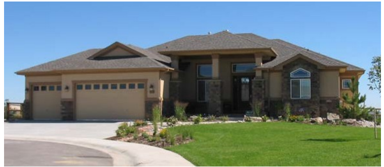
Roof includes a variety of elements including main roof and secondary roofs over porches and pop-outs and includes overhangs
