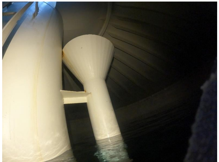
Interior Conditions/Roof Vapor Zone
