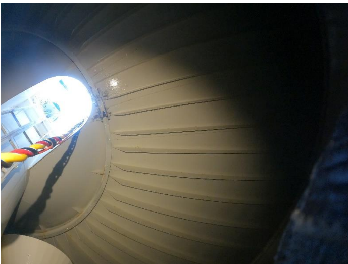
Interior Conditions/Roof Vapor Zone
