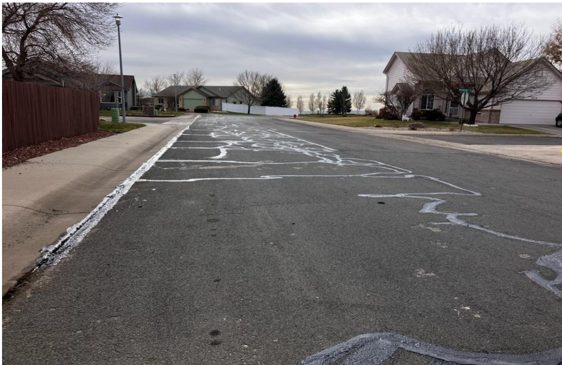
Crack Sealing in The Landings
